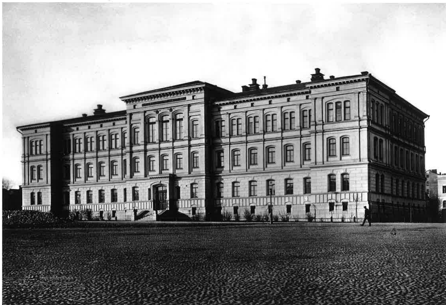
Main building of TKK until 1964.
