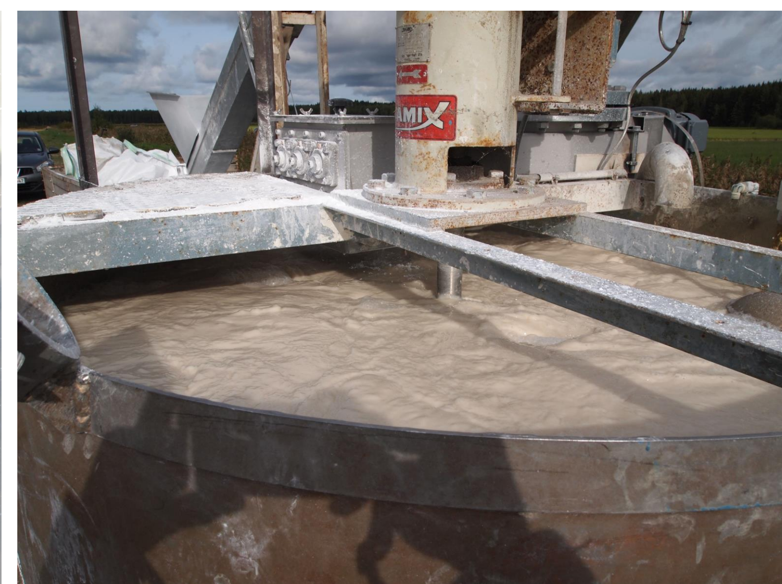
The C2 powder is mixed with river water in a 3 m 3 mixing container
