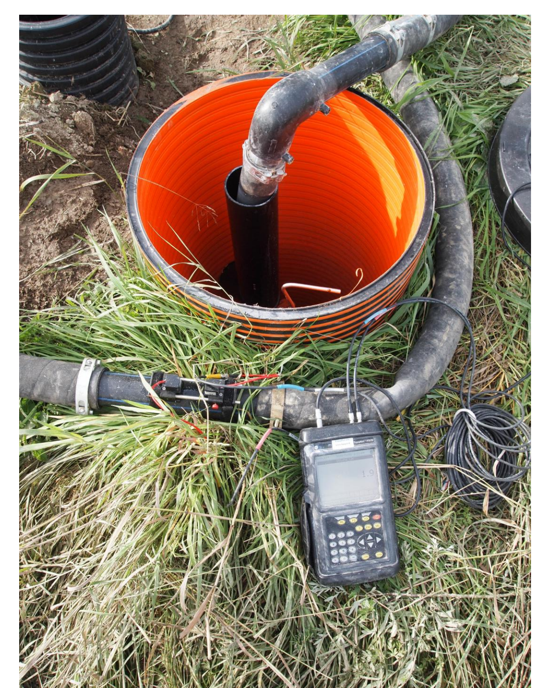
Injection of the suspension into the soil via the injection pipe
